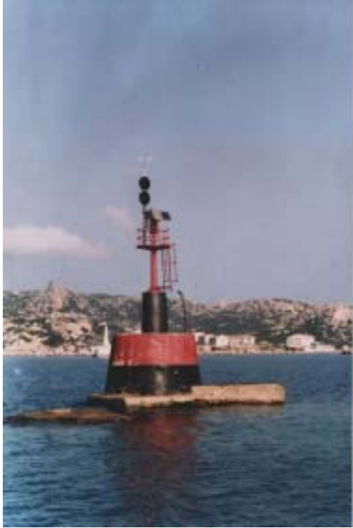
Figure 12-2 The meteorological mast at La Maddalena.
