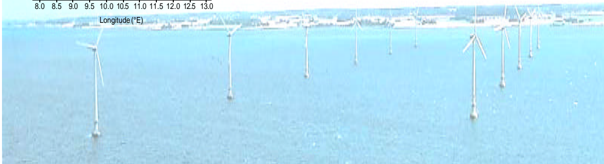
Photo of Vindeby Wind Farm installed in 1991 11 Bonus 450 kW turbines
