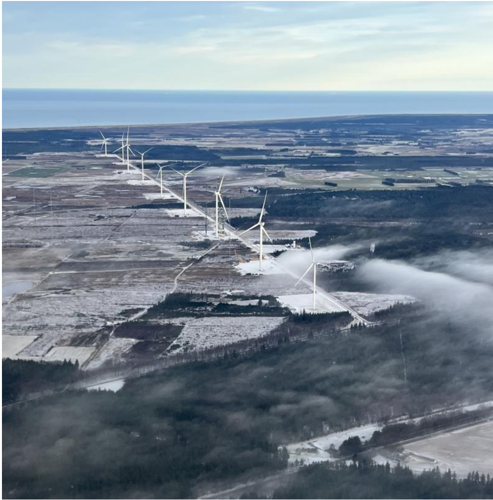
Figure 1: Nine wind turbine stands in Østerild Test Center, Thisted Municipality.
